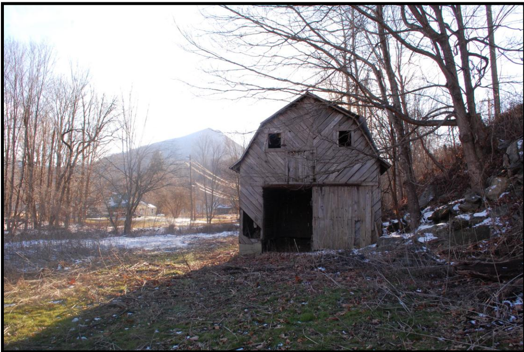
Figure 38: Kelly House Barn, 13943 NC 88, view to the southwest
