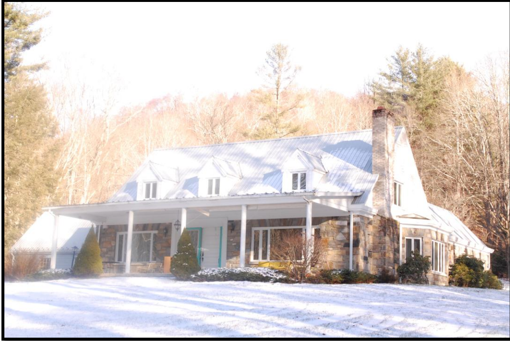
Figure 33: Worth and Mildred Knox House (AH 574), 164 Worth Chapel Road, view to southeast
