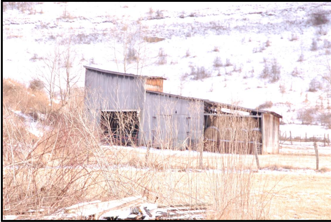
Figure 12: Barn, north elevation, view to southwest
