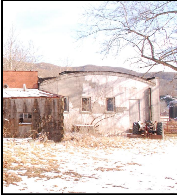
Figure 20: Knox Knitting Mill, north elevation, view to the south-southeast
