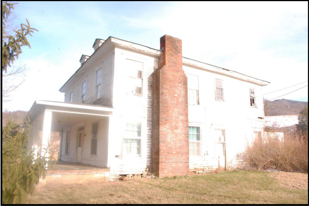
Figure 9: David Worth House, west elevation, view to east-northeast
