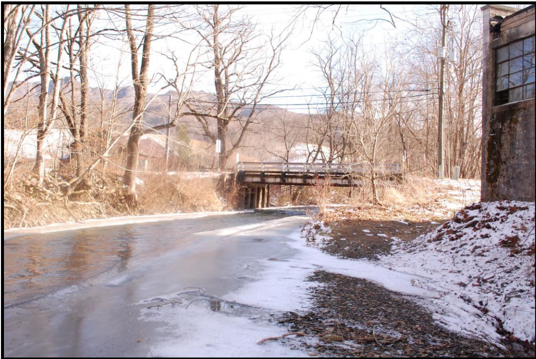
Figure 4: Bridge No 187 on Three Top Road over Tree Top Creek, view to the southeast, Knox Knitting Mill to the right
