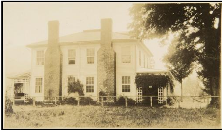
Figure 6: Documentary photo of David Worth House from Ancestry.com (no date), east elevation, view to the west
