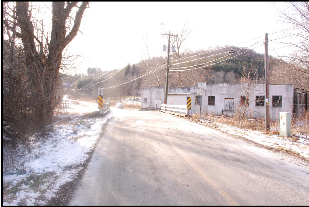
Figure 15: Bridge No. 187 and Knox Knitting Mill (to the right), view to the west
