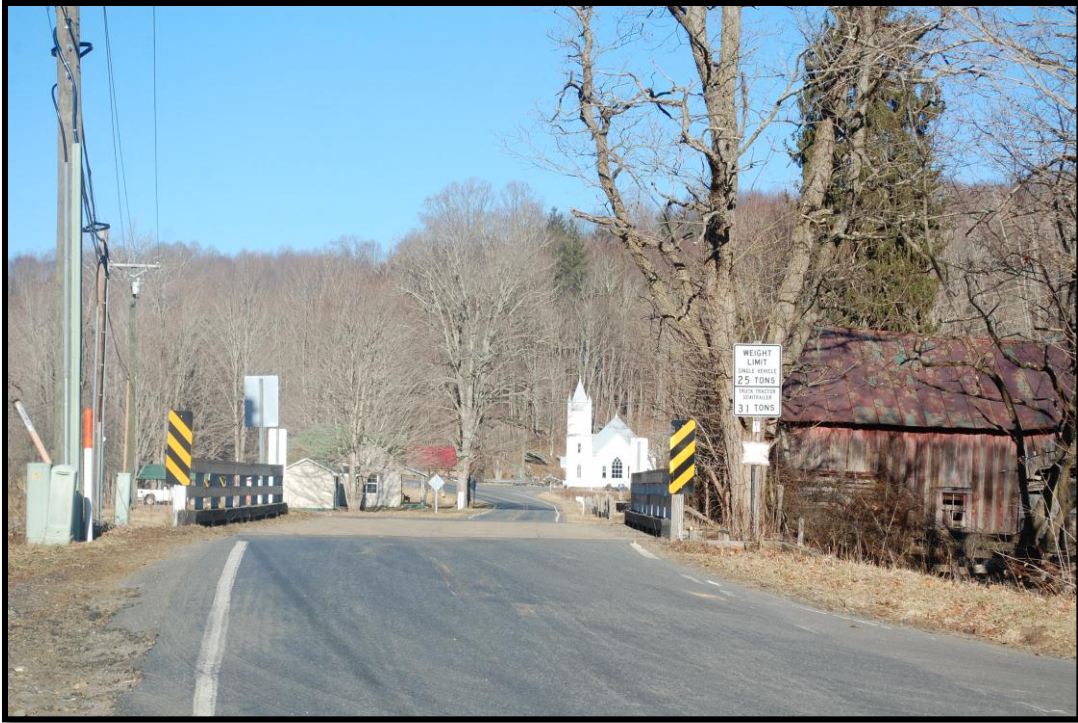
Figure 1: Bridge No. 187 over Three Top Creek, view to the northeast
