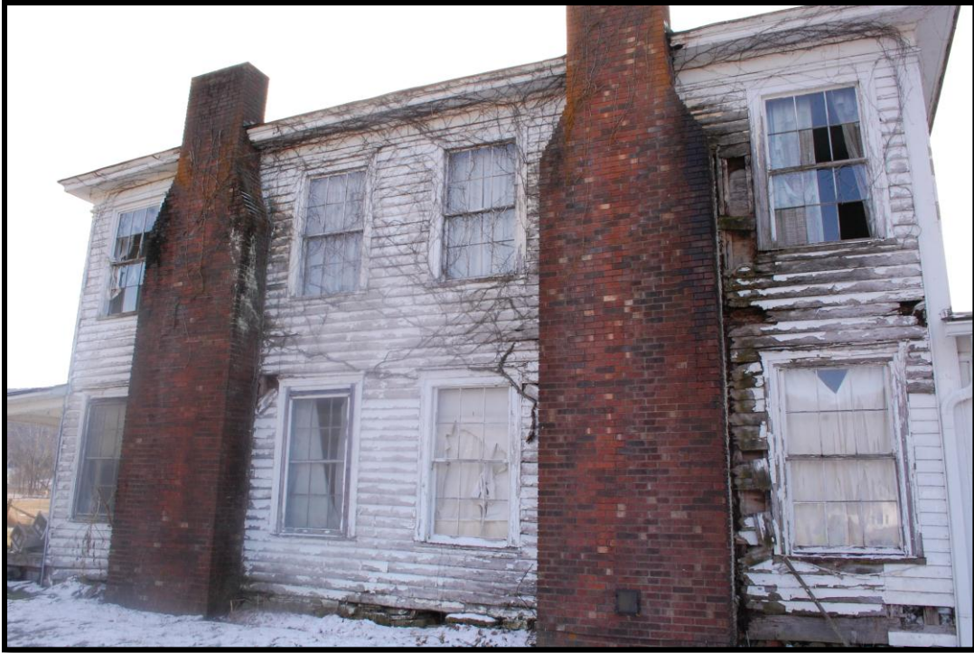
Figure 7: David Worth House, north elevation, view to southwest
