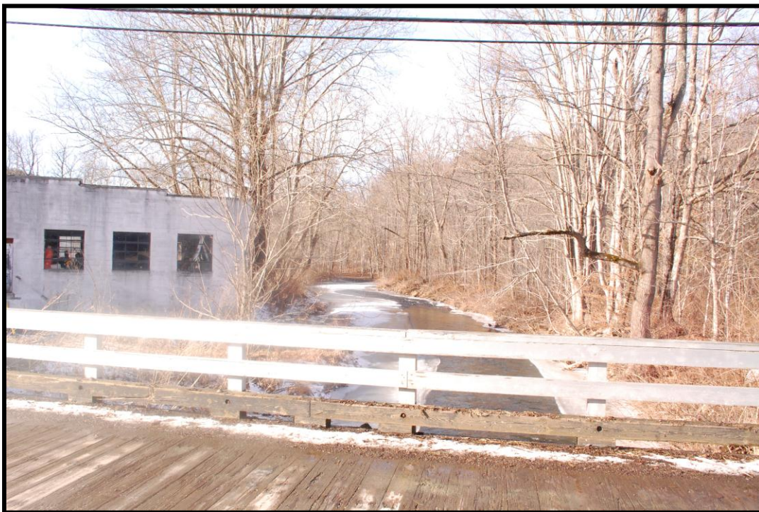
Figure 17: Knox Knitting Mill, eastern section (built 1960), view from Bridge No. 187 to the north-northwest
