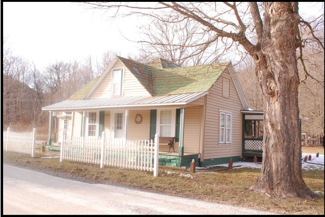
Figure 29: House (AH 321), 292 Three Top Road, view to the northwest
