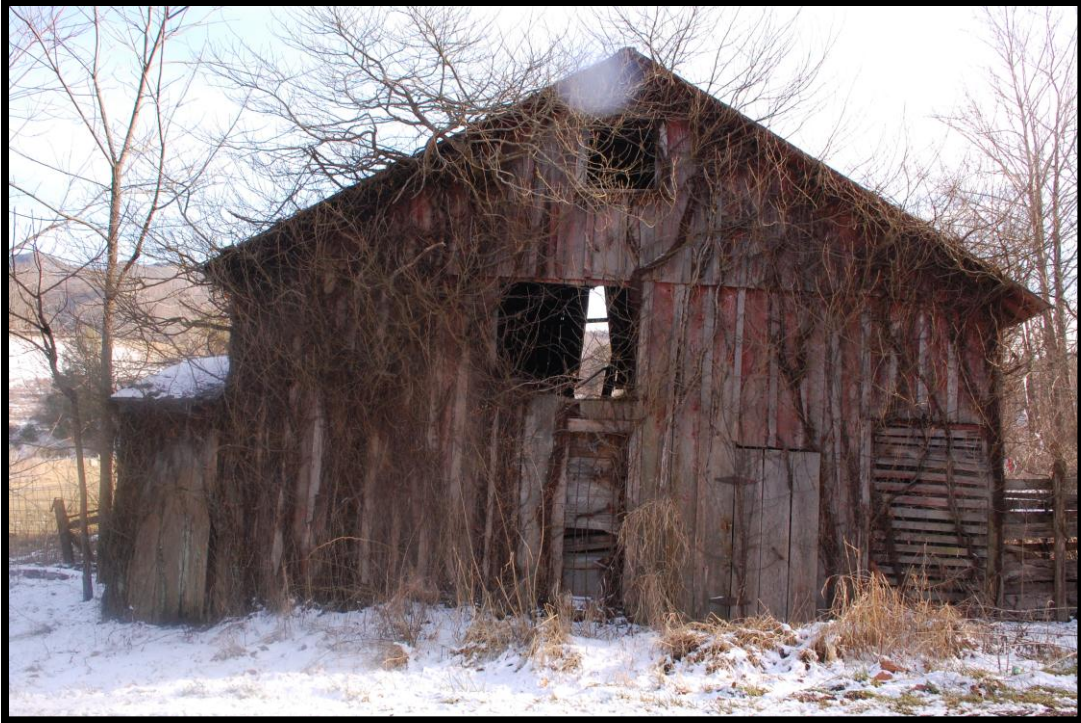
Figure 11: Barn, facade, view to the southeast from Three Top Road
