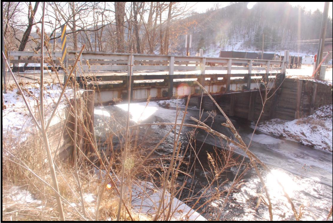
Figure 3: Bridge No. 187 along Three Top Road, view to the southwest
