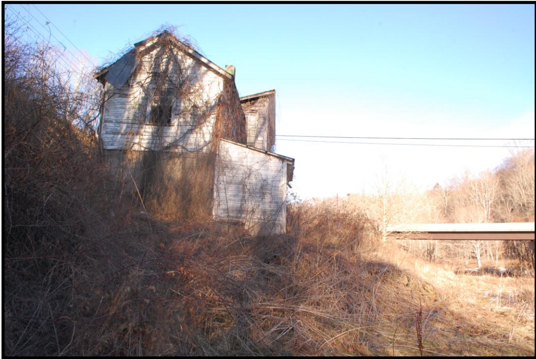
Figure 36: Kelly House, 13943 NC 88, view to the northeast
