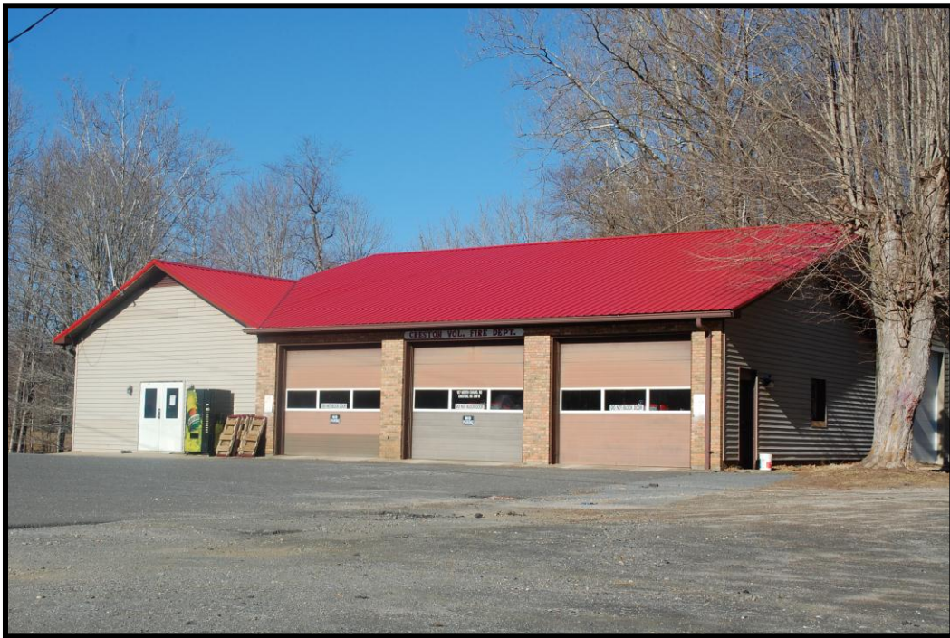
Figure 34: Creston Volunteer Fire Dept., 157 Worth Chapel Road, view to the east-northeast
