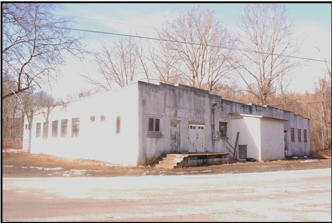
Figure 19: Knox Knitting Mill, southwest corner (1951 section), view to the north
