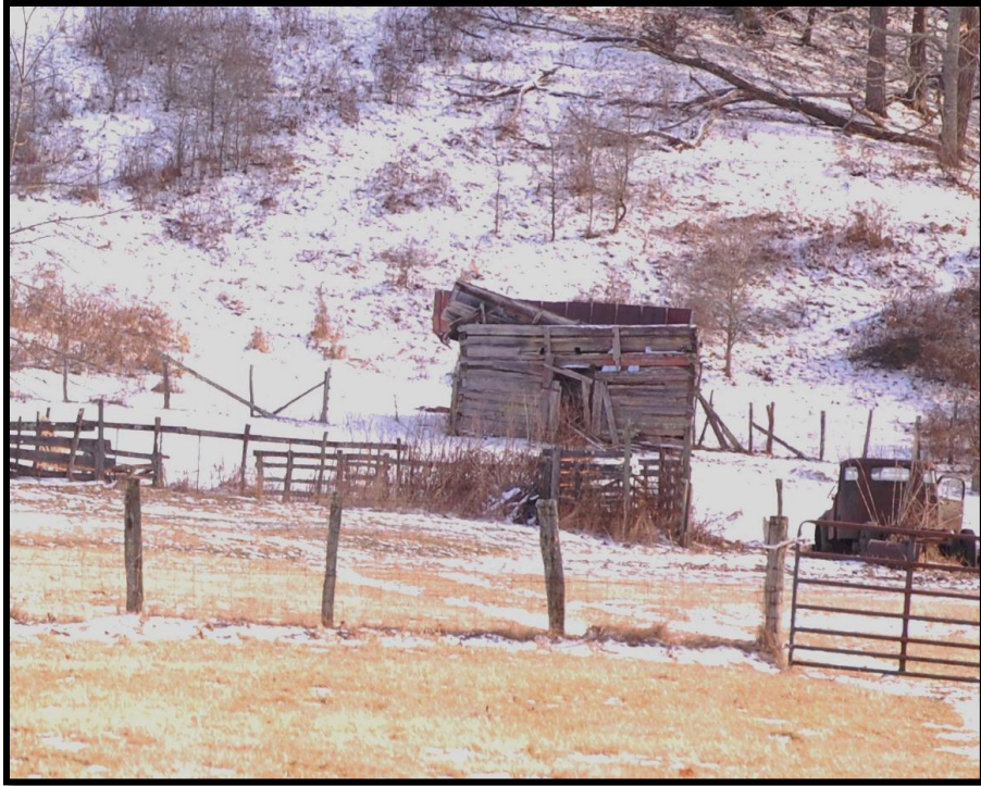
Figure 13: Log building, view to the southeast
