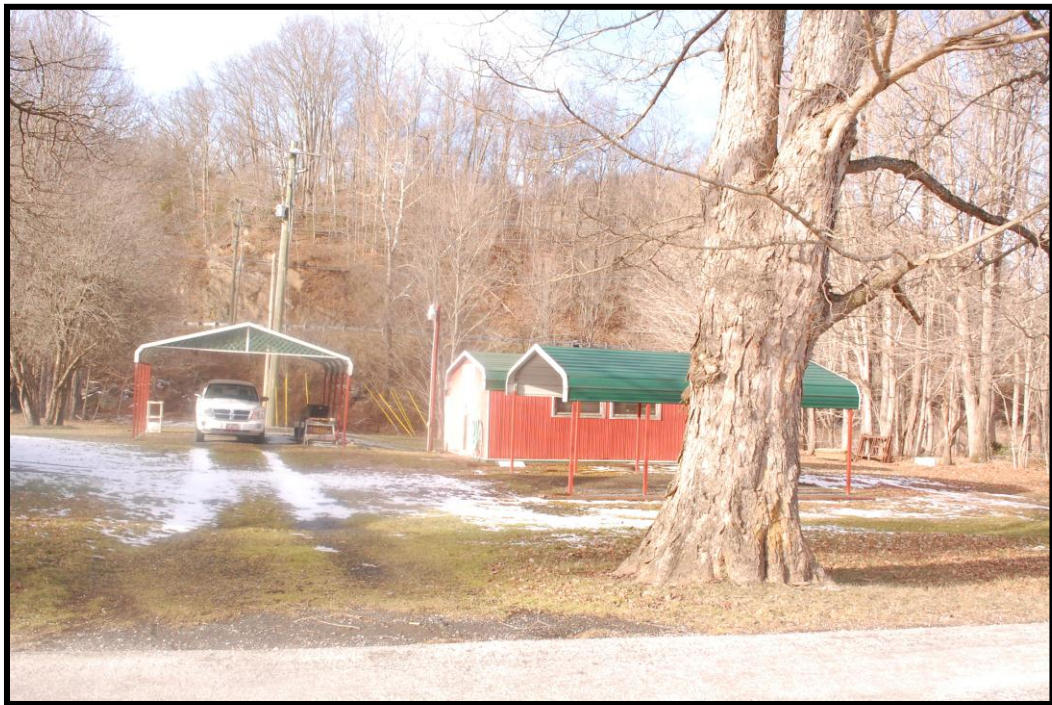
Figure 30: House (AH 321), 292 Three Top Road, auxiliary buildings and structures, view to the north-northwest
