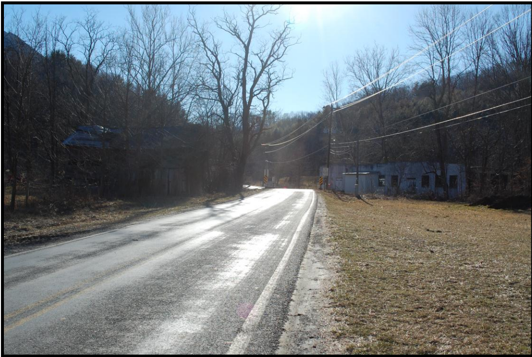
Figure 2: View to the southwest along Three Top Road toward Bridge No. 187
